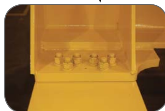
Standard bolted girder connection plates
