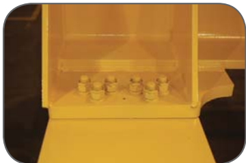
Standard bolted girder connection plates
